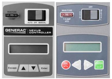
This is the process for resetting a generator when it has a fault code (red light). Before starting to reset the generator, look at the screen that is above the buttons. It will display a fault code and the meaning. Please write down what it says before starting the process. This helps us before coming out to repair if needed.
